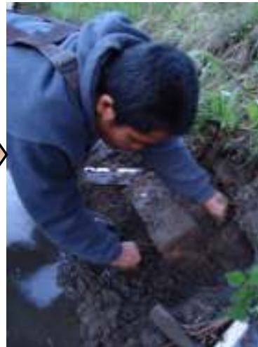
The bottom side was cut using a wire saw.
